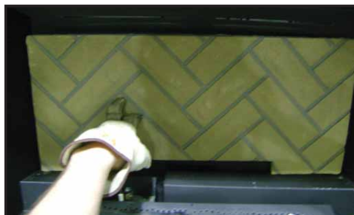
Figure 2. Install Back Refractory
